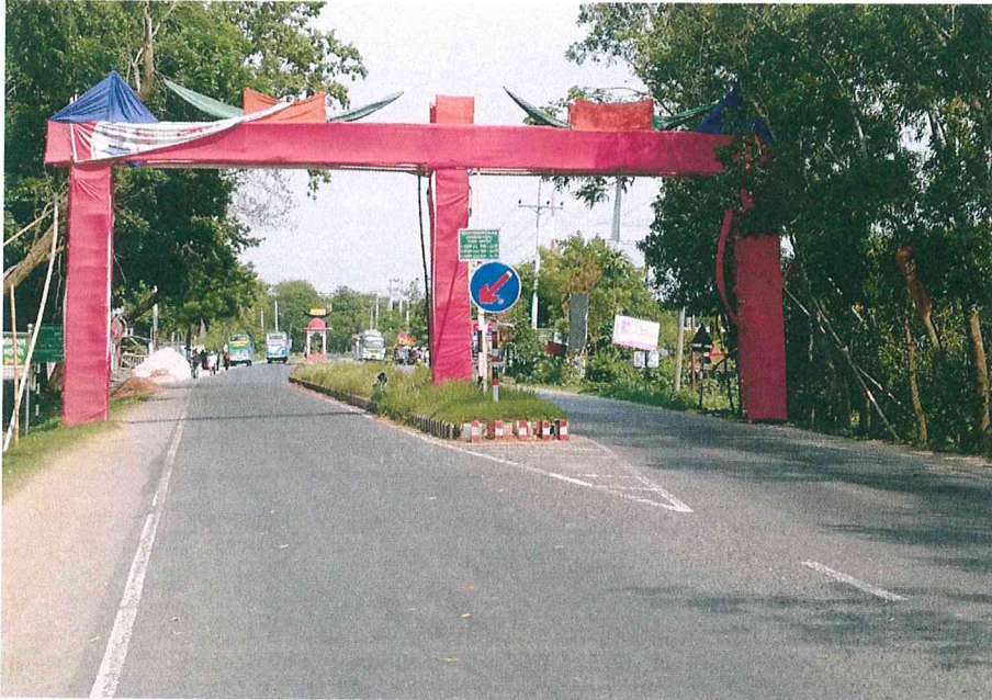
Figure 02d: Unauthorized Structure (Near LRP 038)
