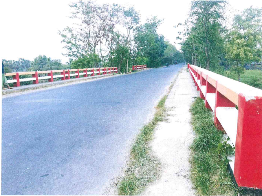
Figure 04c: Bridge (Near LRP 100)
