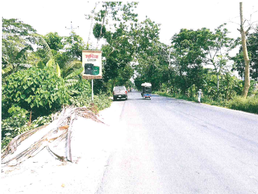
Figure 03b: Unauthorized Billboard (Near LRP 020)
