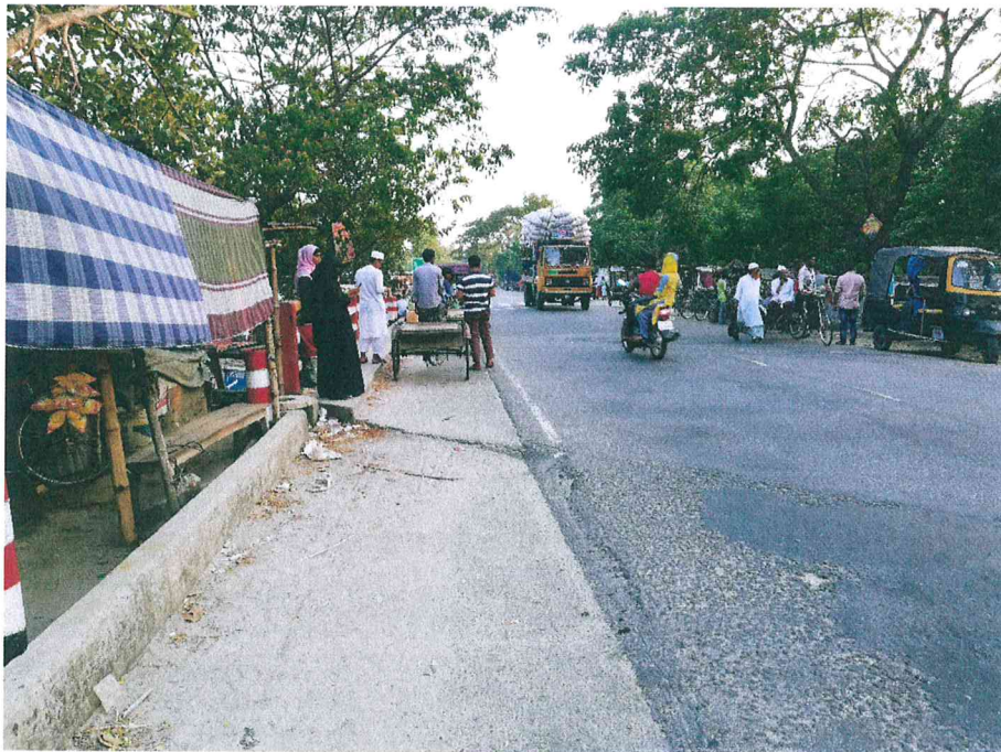
Figure 07 b: Unauthorized Parking & Illegal shops at Bridge site (Near LRP 057)
