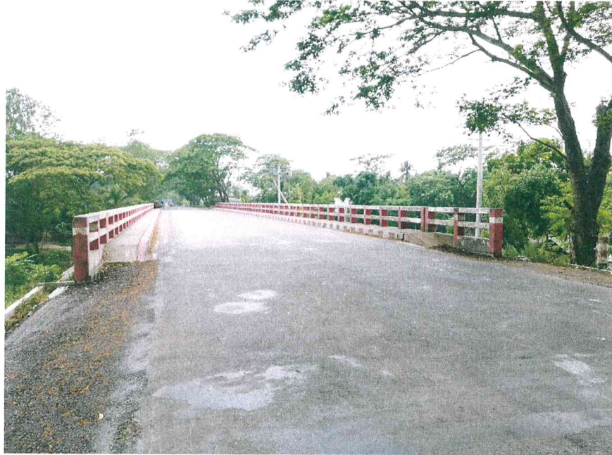
Figure 04a: Bridge (Near LRP 006)
