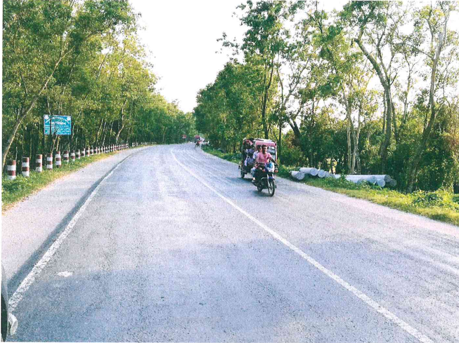
Figure 08: Three wheeler plying on Carriage Way at Sharp Bend (Near LRP 030)
