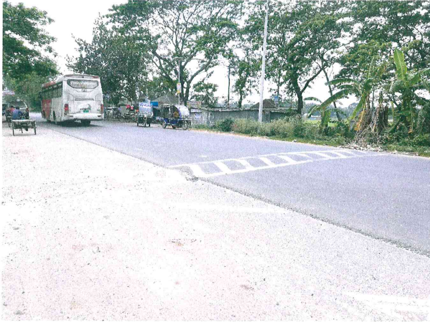
Figure 05a: Unauthorized Speed Breaker (Near LRP 015)
