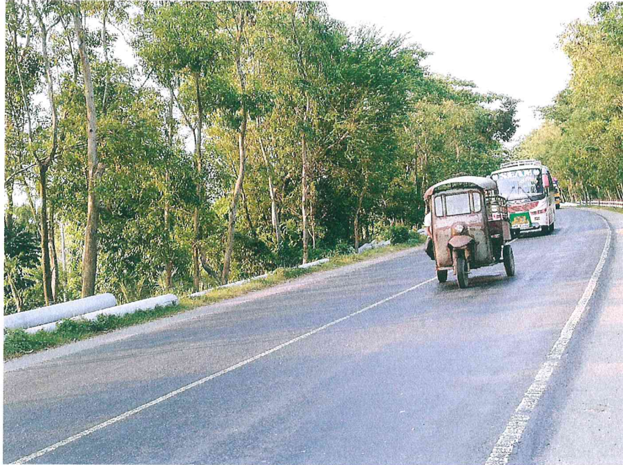
Figure 06c: No road sign at Sharp Bend (Near LRP 030)
