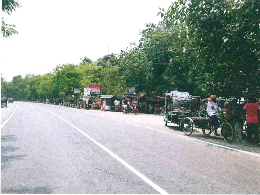
Figure 07a: Unauthorized Parking & Illegal shops at Link Road (Near LRP 022)
