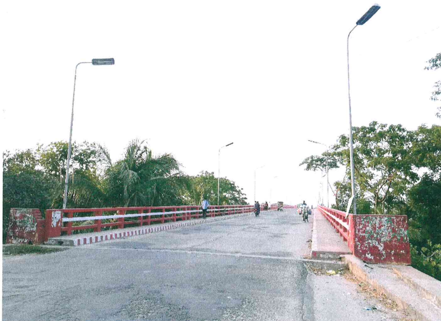
Figure 04b: Bridge (Near LRP 094)
