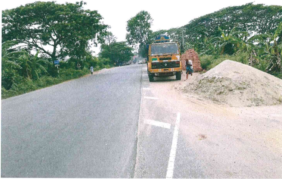
Figure 10: Occupied Bus Bay (Near LRP 013)
